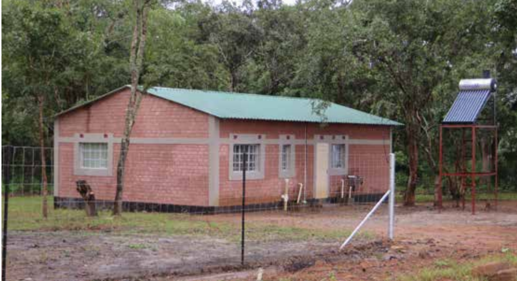
A middle management house at Silverlands Agriculture Services (Kakushi) in Zambia, where all energy requirements are provided by solar power.
