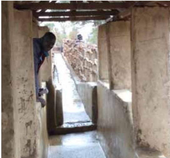
Newly repaired dip station.
