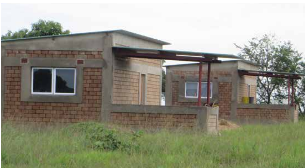
General worker housing at Silverlands Ranching built with hydraform bricks.
