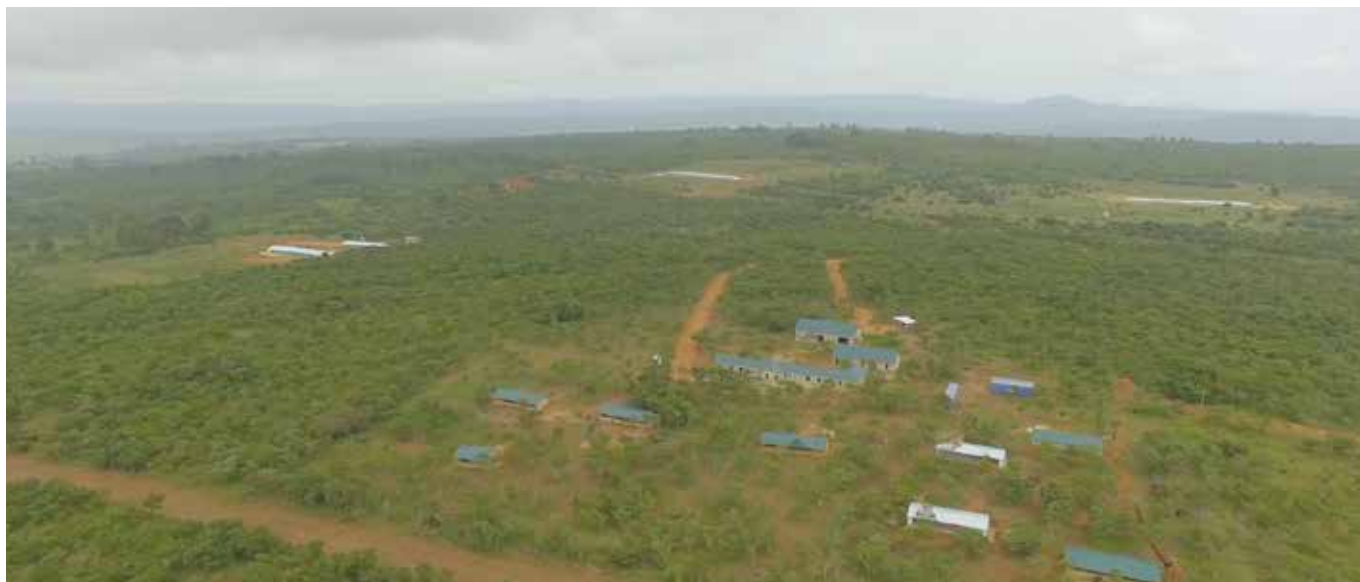
The Poultry Training Centre in the foreground and commercial poultry houses in the distance.
