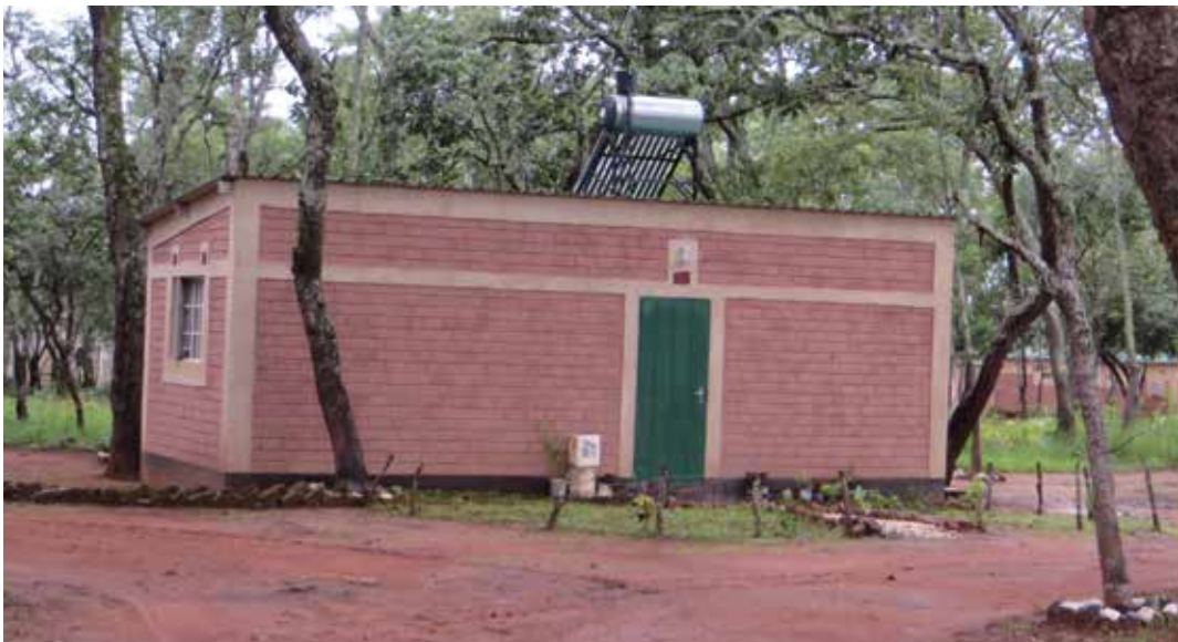
A general worker house at Silverlands Zambia (Serenje). These are arranged amongst the trees in a woodland, with 5 houses sharing ablutions. Housing uses pre-moulded hydraform bricks and designs. The designs are such that general worker houses can be doubled in size in future (hence the lack of windows on the one side).
