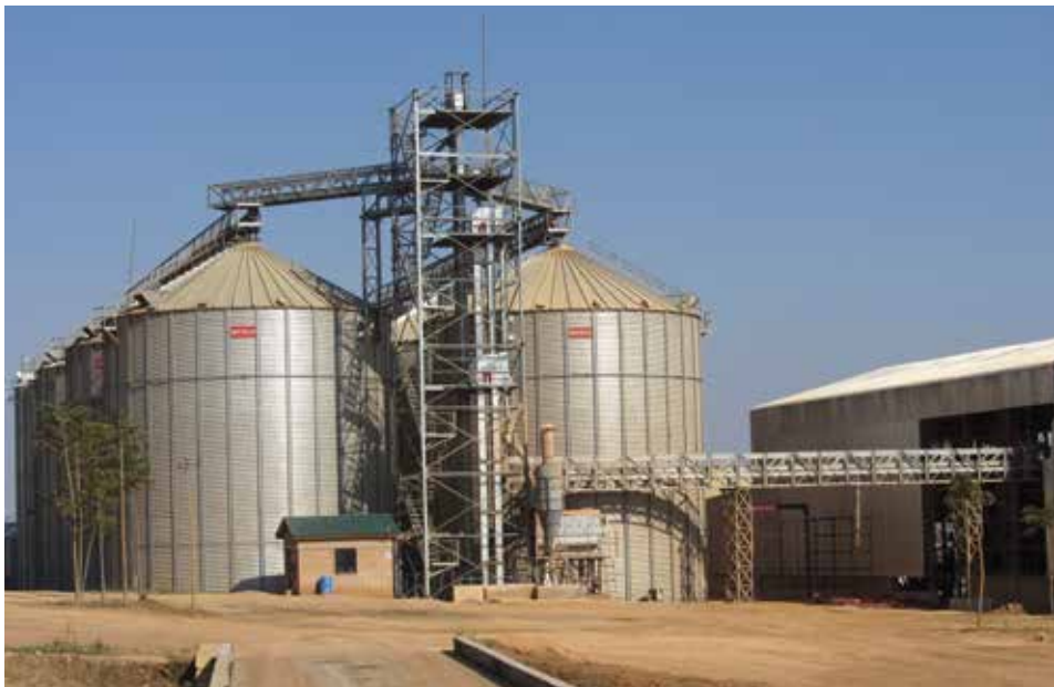
Silverlands Tanzania's hub near Iringa: the weighbridge leading to 32,000 t of silo storage and new 40 t/hr feed mill housed on the right.
