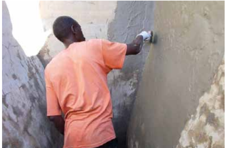
Repairing a dip station.
