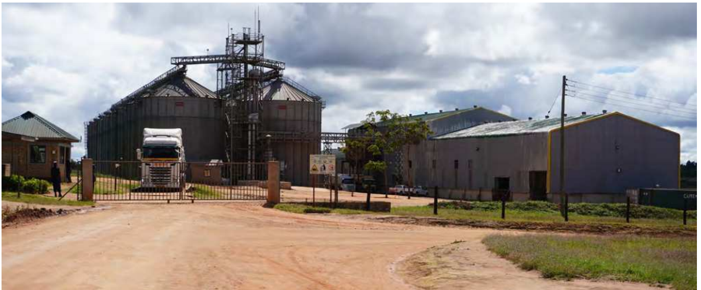
Silverlands Tanzania: Silo storage complex and feed mill built as part of this development.
