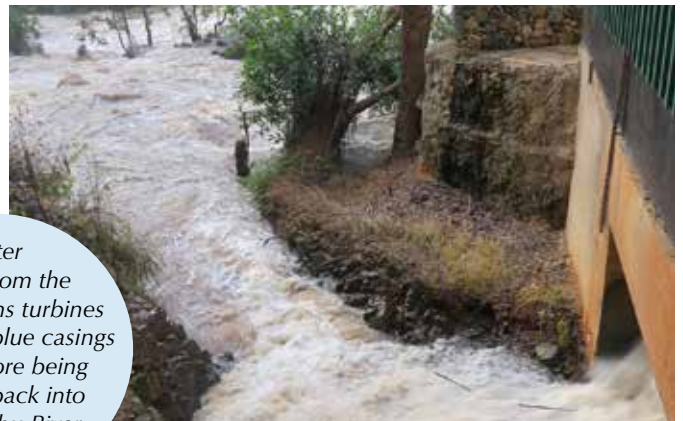
Silverlands Ndolela is privileged to have use of an 80m drop on the large Ruhuhu River (left) – the perfect location for a hydropower plant. A small quantity of the total river volume flows into a pipe that drops steeply down a bank and into the turbine house (right).
