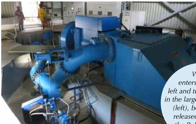
Silverlands Ndolela is privileged to have use of an 80m drop on the large Ruhuhu River (left) – the perfect location for a hydropower plant. A small quantity of the total river volume flows into a pipe that drops steeply down a bank and into the turbine house (right).
